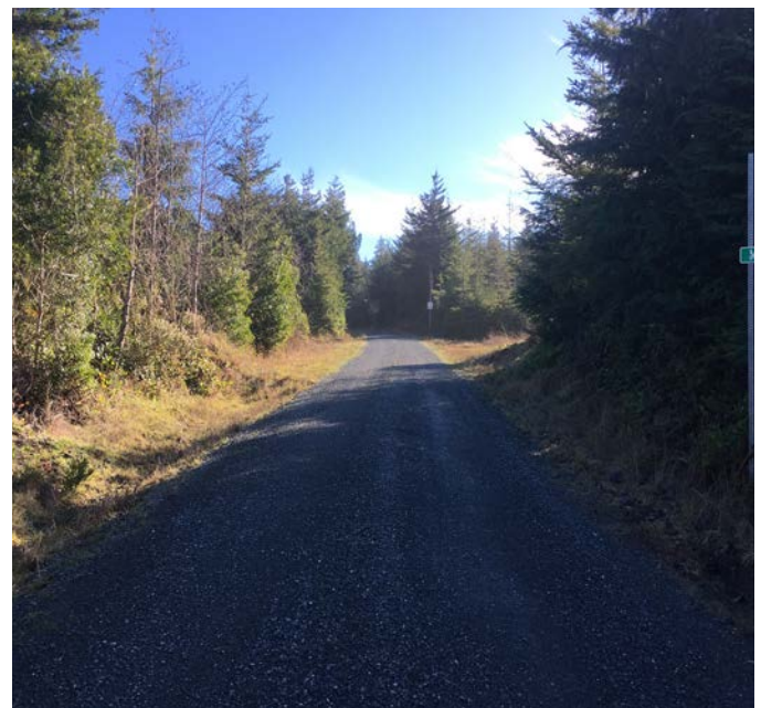
Miluk Extension looking southeast
