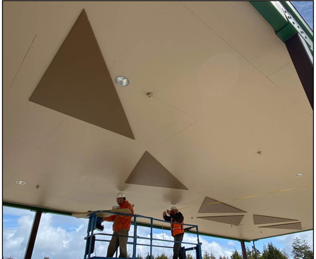
Workers attach decorative triangles to the underside of the porte cochere's cover at the main entrance. The triangles mimic a traditional basketry design element.
