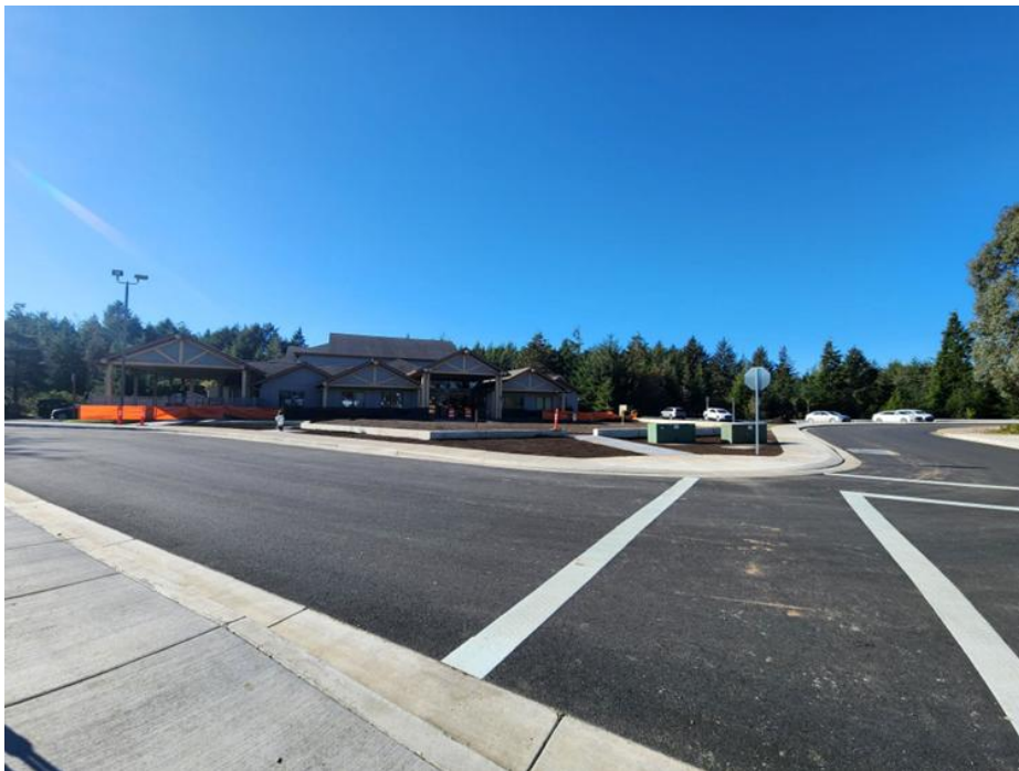
Figure 10. Completed “Tee” Intersection at Miluk Drive and Mexeye Loop (2023)
